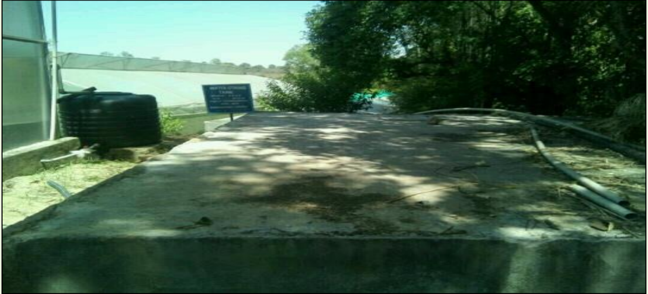
Water storage Tank
